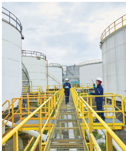
Driven by operational excellence, our plant and terminals continue to deliver flawless operations to ensure seamless terminal throughput and delivery
