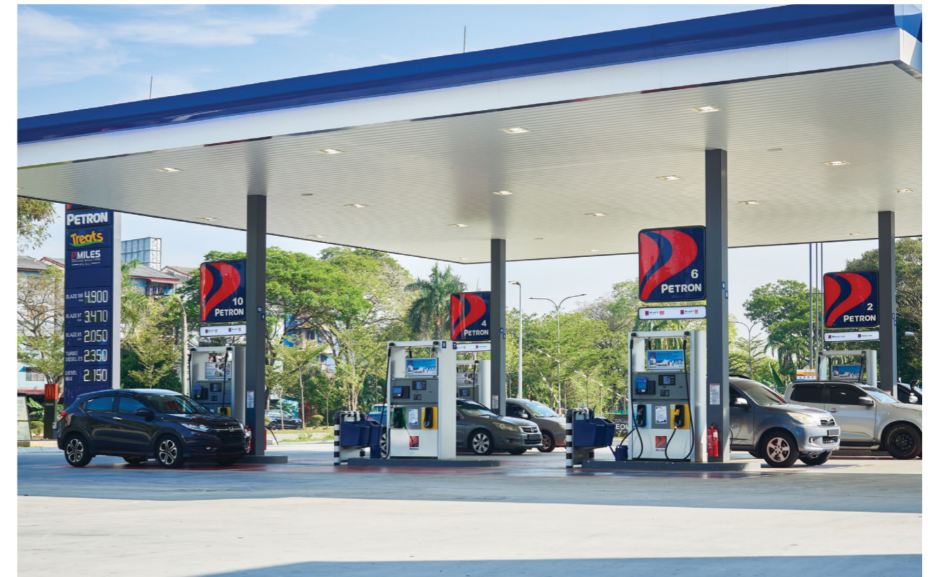
The service station is fitted with energy efficient LED lightings under the canopy
