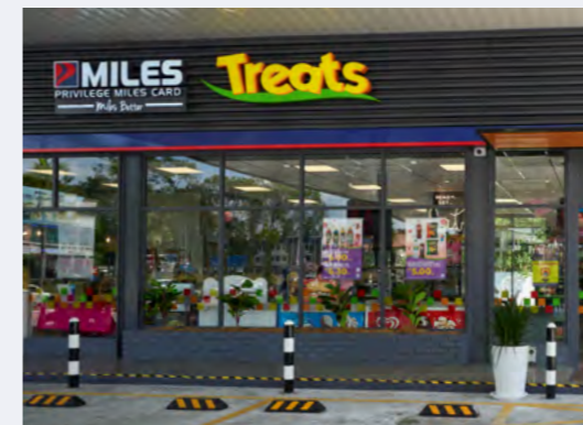
Our new service station design with a medium-sized Treats store in Petron Seremban 2.
