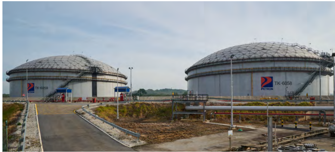
The successfully commissioned MIF2 with the two new 250,000-barrel products tanks contribute savings in logistics cost.
