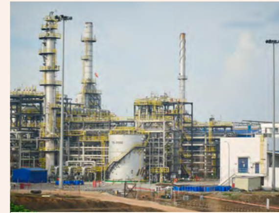
The new DHT facility enables us to process ultra-low sulphur automotive diesel. This is in compliance with Government's mandate to introduce Euro 5 specification diesel.
