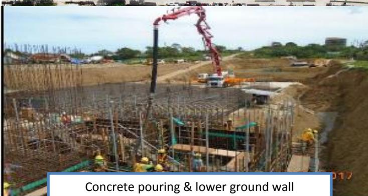
Concrete pouring & lower ground wall
