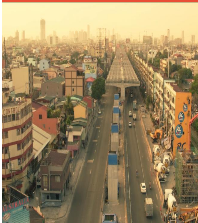
Ongoing works on Section 3
